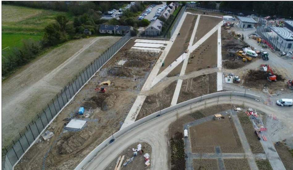
Figure 5: Horticulture area created using arisings from the works to optimise vertical orientation for capturing higher levels of sunlight
