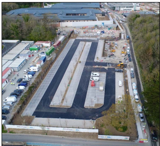
Figure 6: Permeable paving carpark serving the proposed facility providing 255no. parking spaces for staff and visitors.
